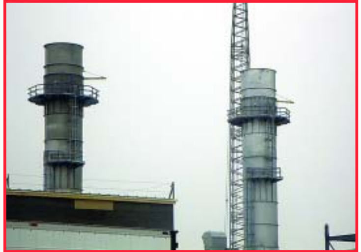
ACCIDENT FREE: Attention to safety pays off at the Salt Valley Generation Station work site, which has remained accident-free despite difficult conditions.
