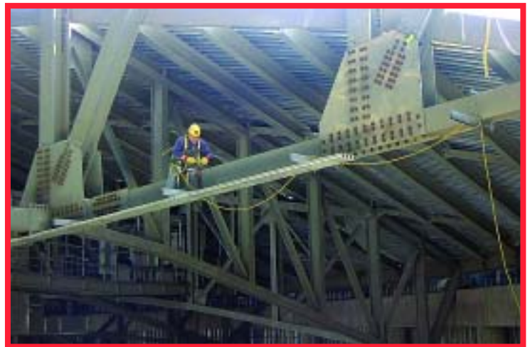
HIGH WIRING: Phil Bremkin connects an electrical conduit high atop the new Omaha Arena and Convention Center.
