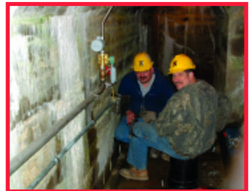
Ron Castro & Buzz Dicks Installing Conduit in Observation Tunnel at Columbus Site
