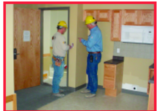
Curt Glass & Steve Wilken Checking Suite Entry Switching
