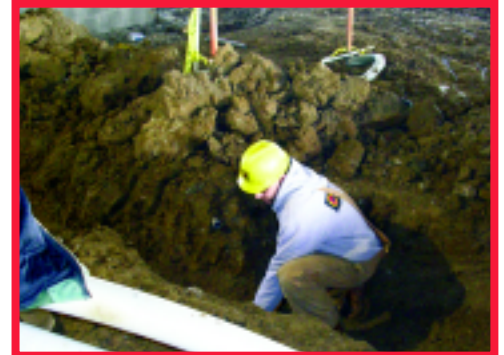
Kirk Cosaert Installing Panel Service Feeders
