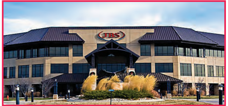
JBS Swift Plant
