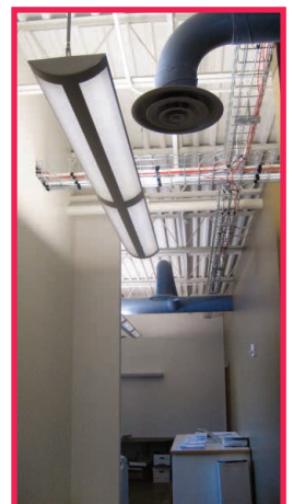
Interior Office Space
