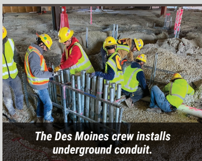
Phase 1 of the new DSM airport terminal.
