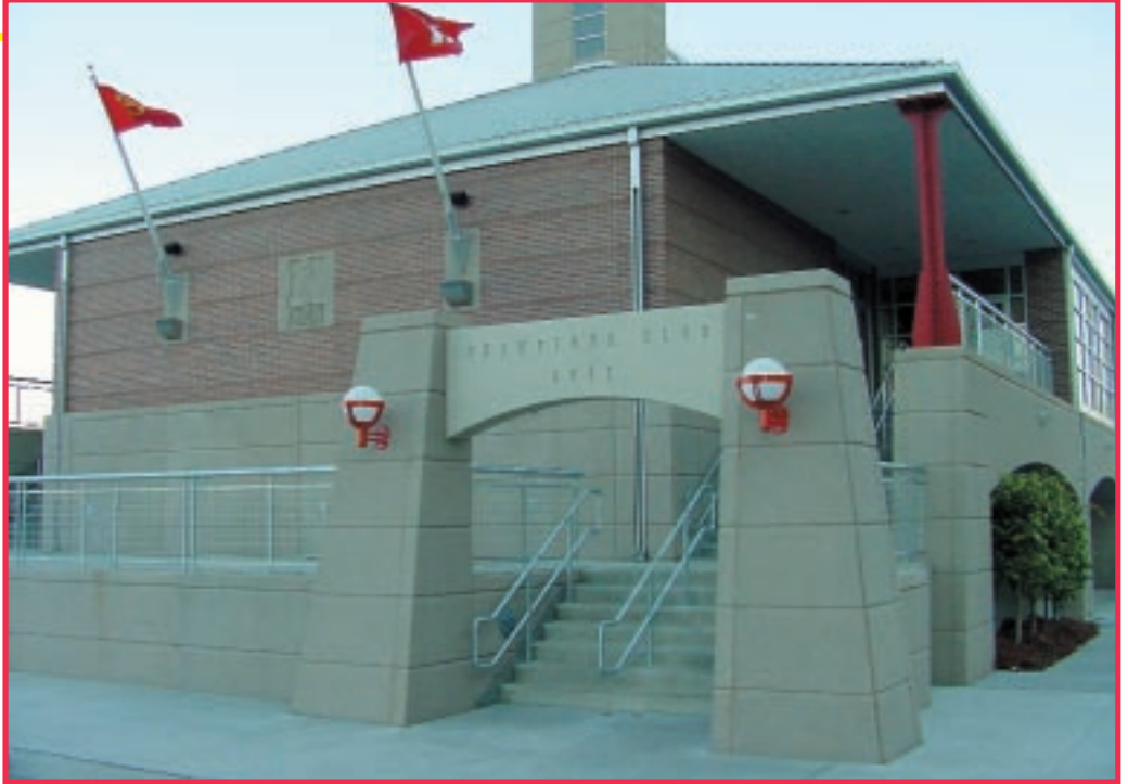
Above: Commonwealth Electric was selected as the electrical contractor for the University of Nebraska Alumni Association's newly-completed Champion's Club.
