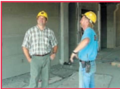
Above: Superintendent Troy Bear and Project Manager Bob Philipps inspect the work at the University of Nebraska Alumni Association's new facility.
