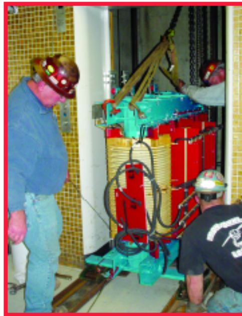
3rd Floor move 750KVA XFMR into shaft
