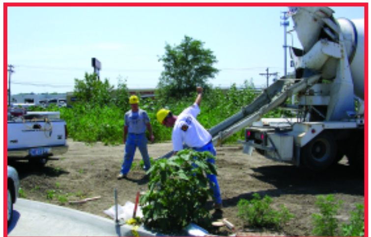
Superintendent Jason Rieckman and Kris Swanson Pouring Pole Bases
