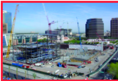
Construction of Phase 2 of Phoenix Convention Center
