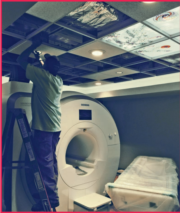
Robin Pearson, Project Foreman, working on the VA MRI project
