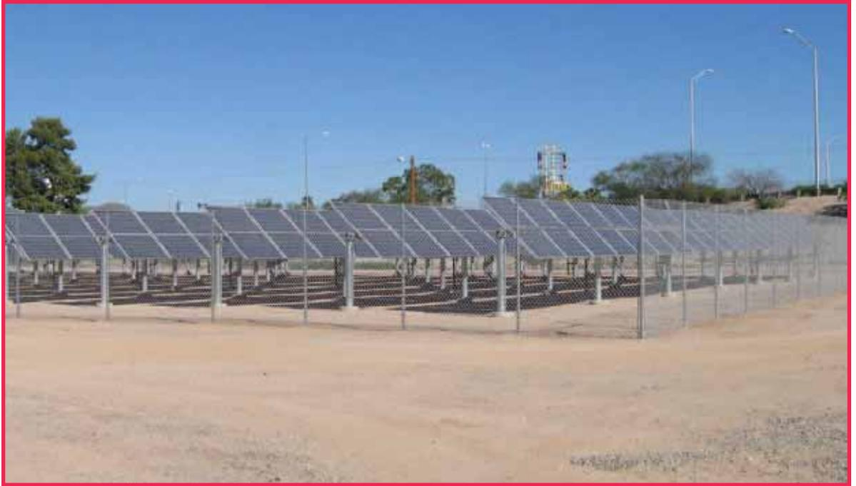
The carport solar project is the second solar energy project that CECM has teamed up on with REC Solar at the Tucson VA Hospital. This new project comes on the heels of the recently completed 302 kW single-axis, tracker system that follows the sun during the day for maximum efficiency. This system, which was completed in May, is the first of its kind at a VA facility nationwide.
