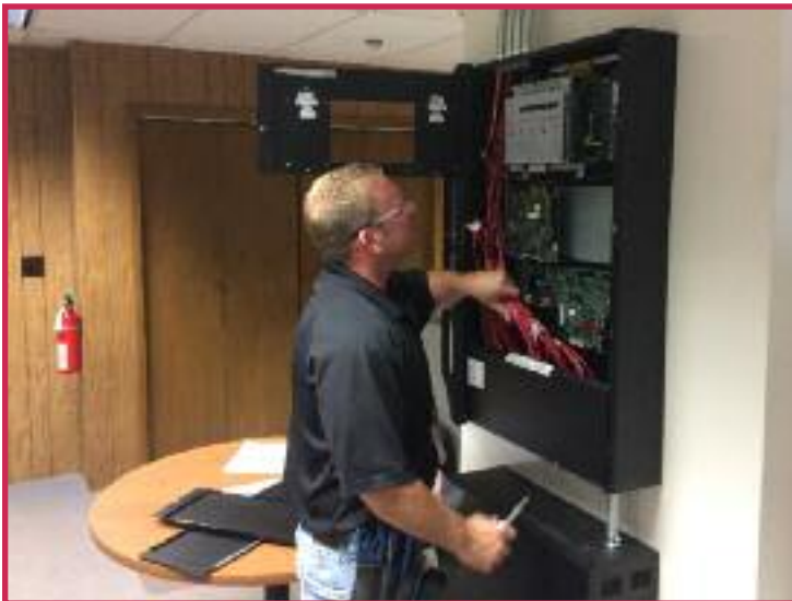
Derek Smith, Technician, performing panel terminations.
