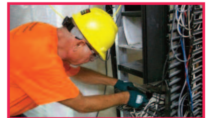
Demo of Existing Closet
