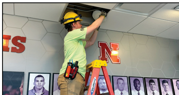
A member of the Lincoln team installs a new wireless access point inside UNL's Memorial Stadium.
