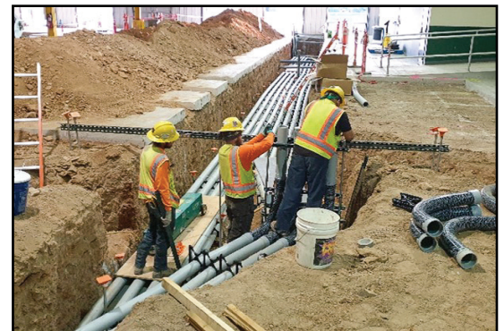
The Tucson team installs underground feeders.
