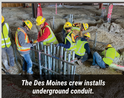
Phase 1 of the new DSM airport terminal.
